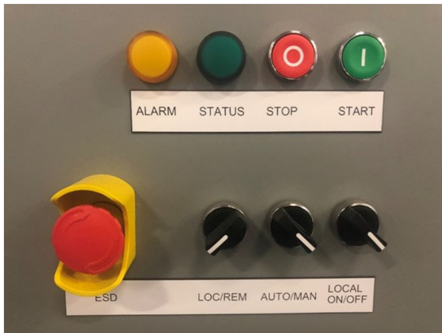
Figure 6-1 – Operation Switches
