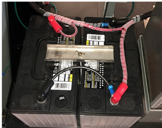
Figure 4-6 – Batteries and Connectors
