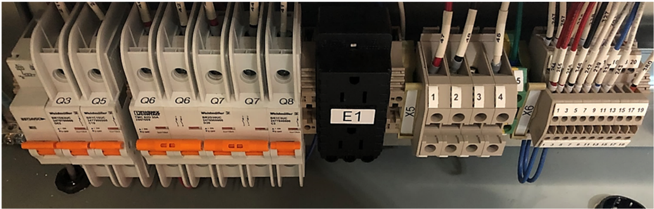
Figure 5-3 – Breakers Located Inside the Electrical Panel Enclosure (Single Phase)
